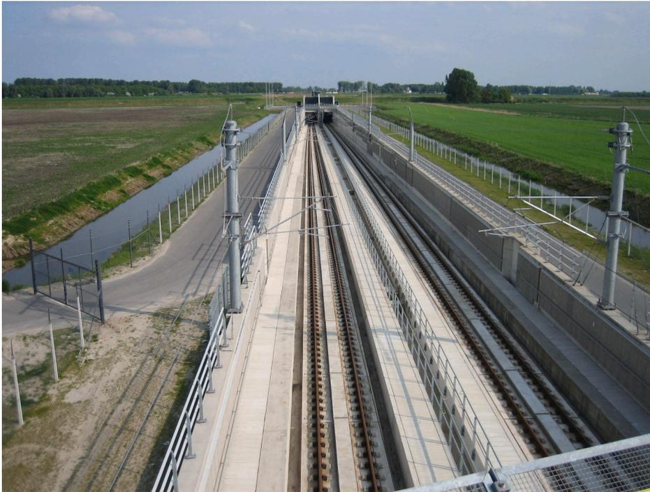
Fig. 42. A ballast-less track between rail tunnels under a river in the Netherlands. Reproduced under CC BY-SA 3.0, <https://creativecommons.org/licenses/by-sa/3.0/deed.en>, courtesy of Hullie.
